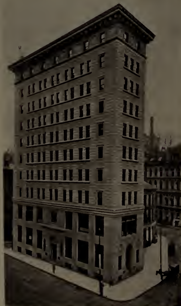
WORTHINGTON BUILDING, State Street.
